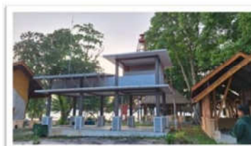
Tsunami Early Warning System
